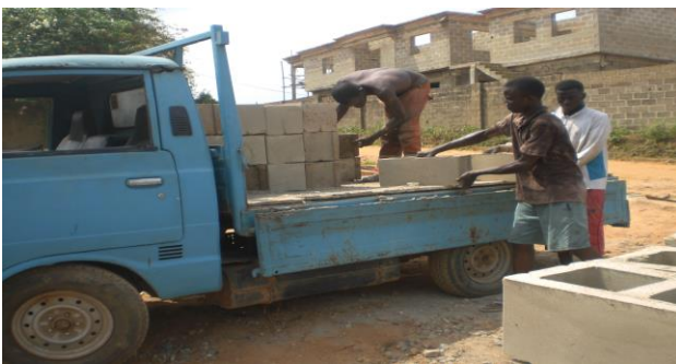
Figure 9: Offloading blocks for use on site.
