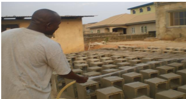
Figure 7: Wetting of blocks at curing section.
